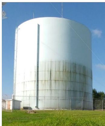
BEFORE: Thermocline Line Visible on Outside of Tank
