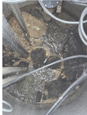
Mandeville Lift Station 27 two days after installation
