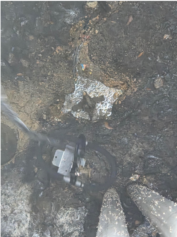
Mandeville Lift Station 27 HydraForce™ by Kasco® installation
