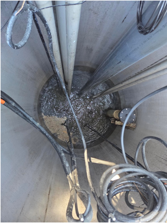
Mandeville Lift Station 27 two weeks after installation
