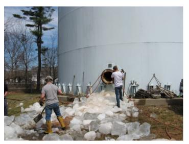
As temperatures continue to drop, ice can form both inside and outside the tank. Each cycle of rising and falling water levels contributes to the formation of ice collars, which become thick and heavy, potentially damaging the tank's integrity.
